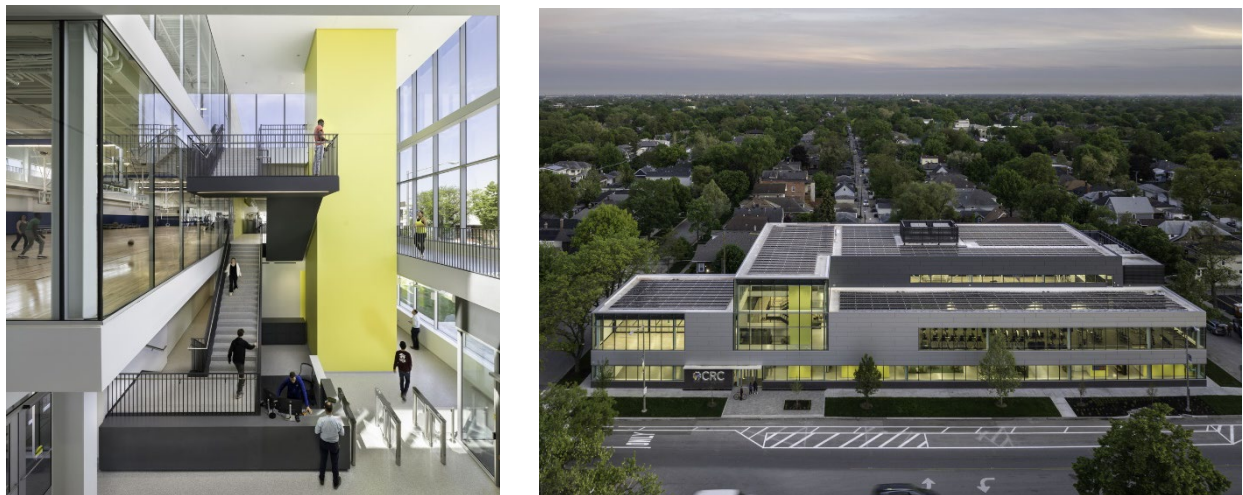
Figure 3.9 Oak Park Community Center (Perkins&Will, 2023)
