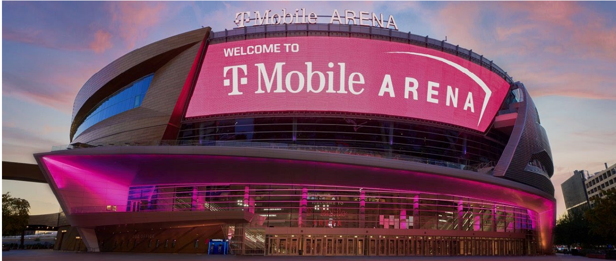
30 - T-Mobile Areana Facade - https://www.t-mobilearena.com/arena-information
