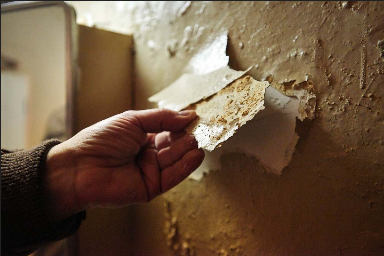
Keivom, J. Gov. Andrew M. Cuomo of New York examined peeling paint in a NYCHA apartment in 2018. [Photograph]. New York Times.
