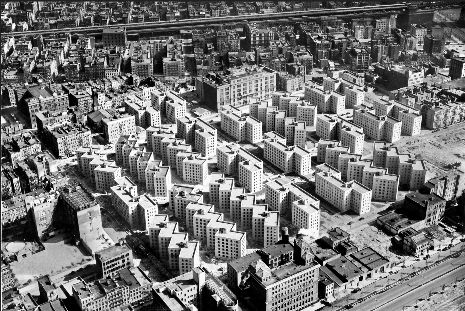
Arnold & Kellogg, The Vladeck Houses, built in 1940 on Manhattan's Lower East Side, were a series of six-story plain brick buildings with generous open spaces. [Photograph, New York Times.]
