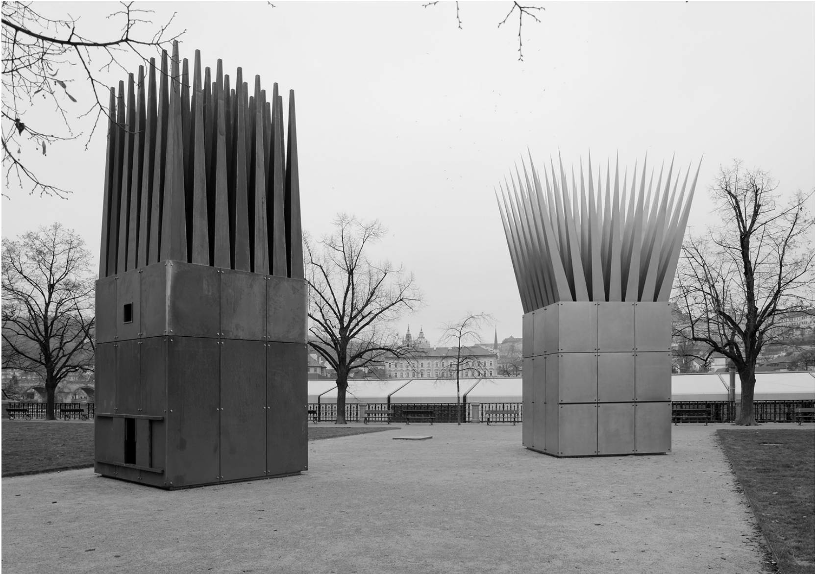
The House of the Suicide and the House of the Mother of the Suicide by John Hejduk
