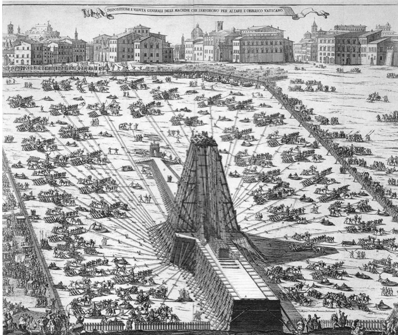
Construction site of the Vatican obelisk at St. Peter's Square by Carlo Fontana
