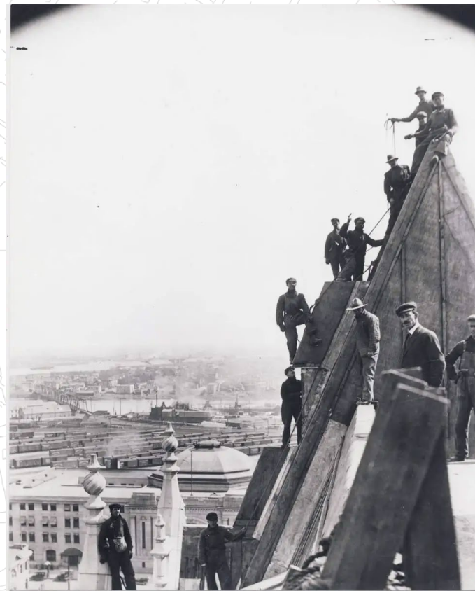
Builders installing the roof of the Fort Gary Hotel 1912
