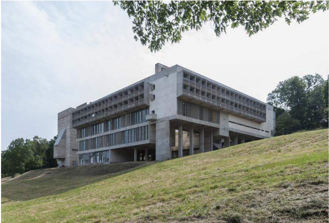
Figure 3.5. La Tourette (Arch Daily 2010).
