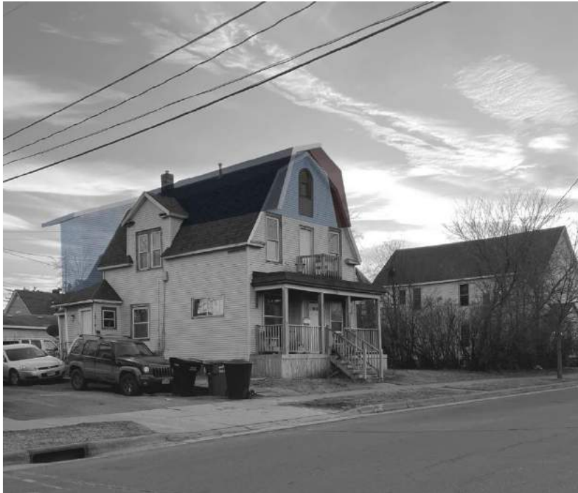
Figure 4.61. Apartment Addition 1214 N 12 th St, Superior WI.
