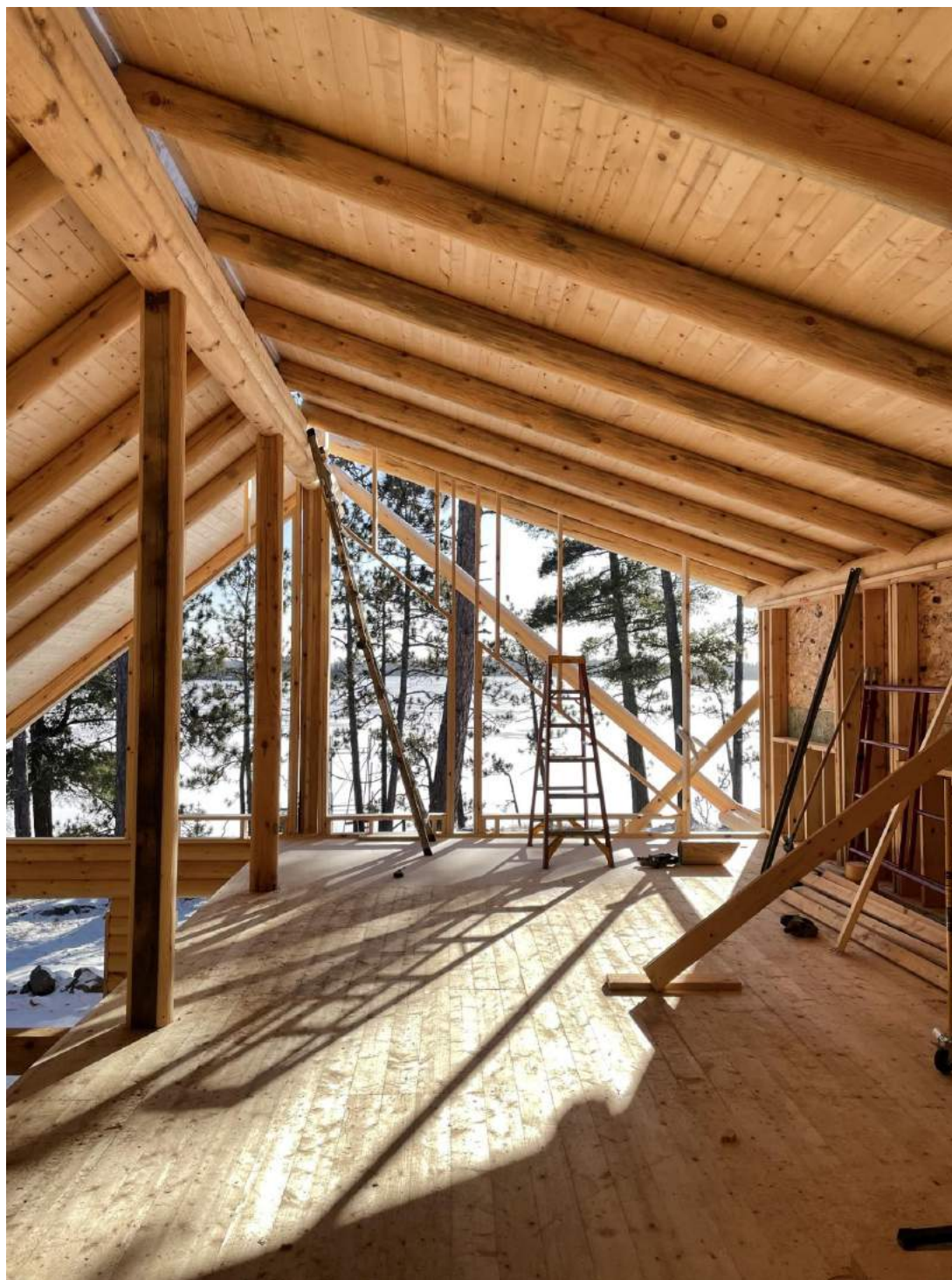
Figure 3.22. Loft Inside Log Cabin
