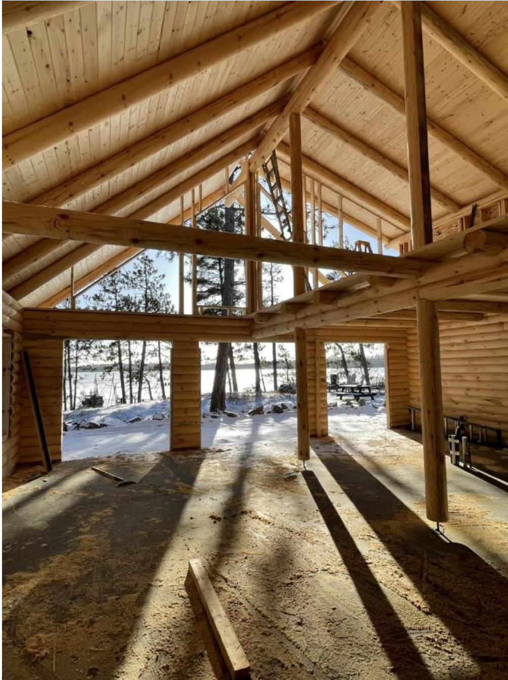
Figure 3.19. Inside Log Cabin Looking Outside.
