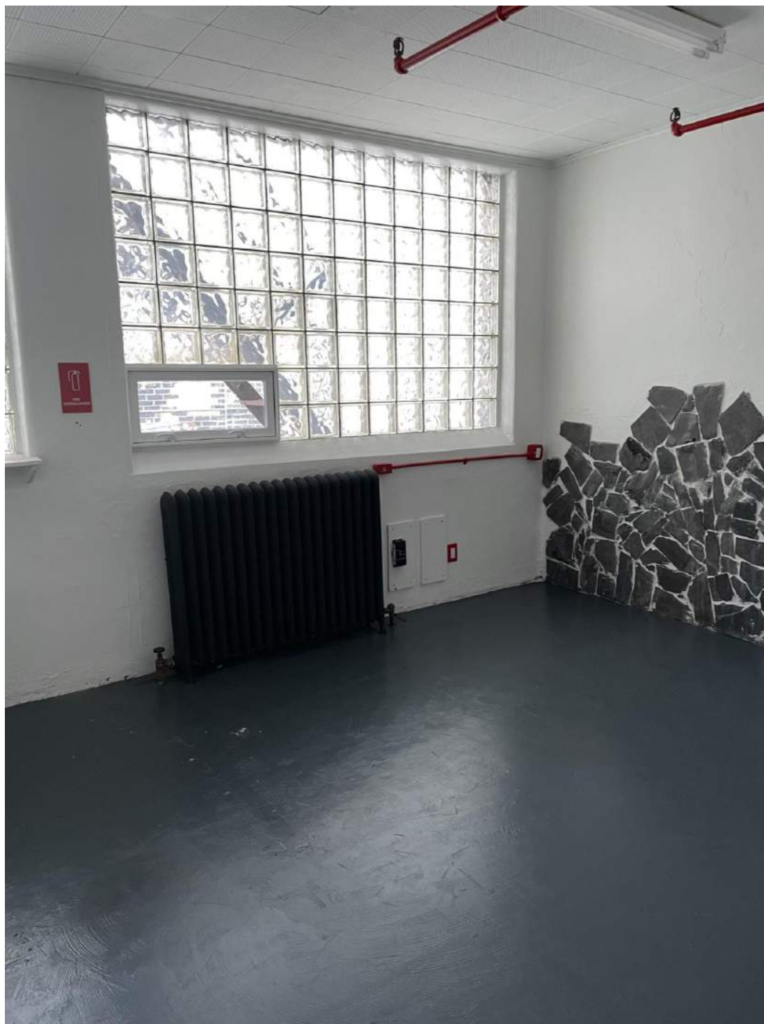
Figure 4.43. Lower Level Office 18W 1 st St, Duluth MN.
