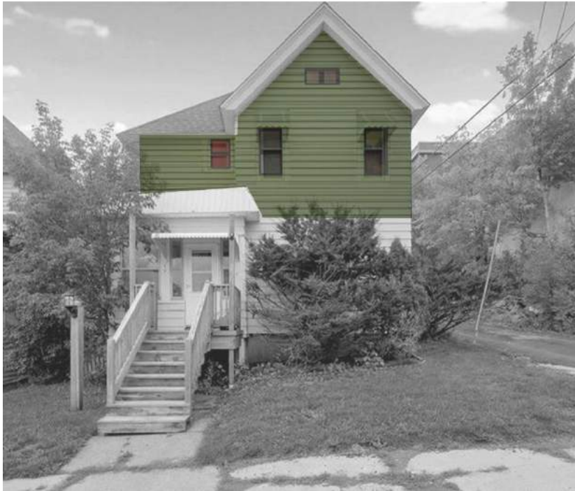
Figure 4.57. Apartment Addition 513 N 2 nd Ave E, Duluth MN.
