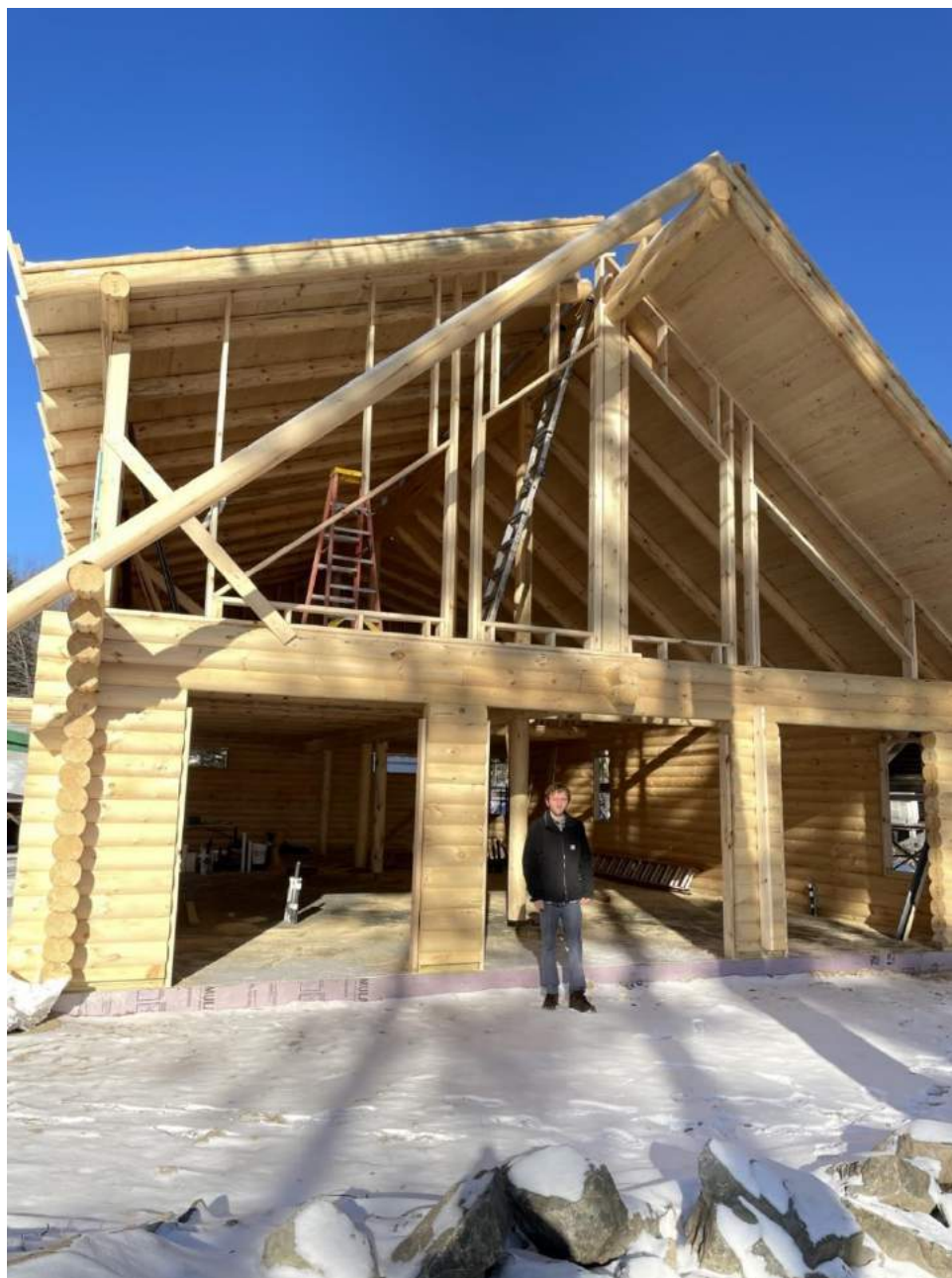
Figure 3.23. Outside of log Cabin.
