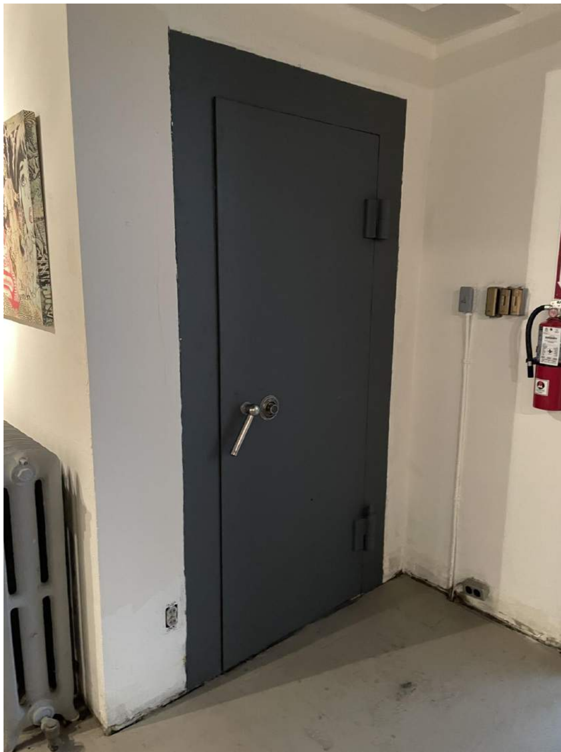
Figure 4.44. Lower Level Old Safe 18W 1 st St, Duluth MN.
