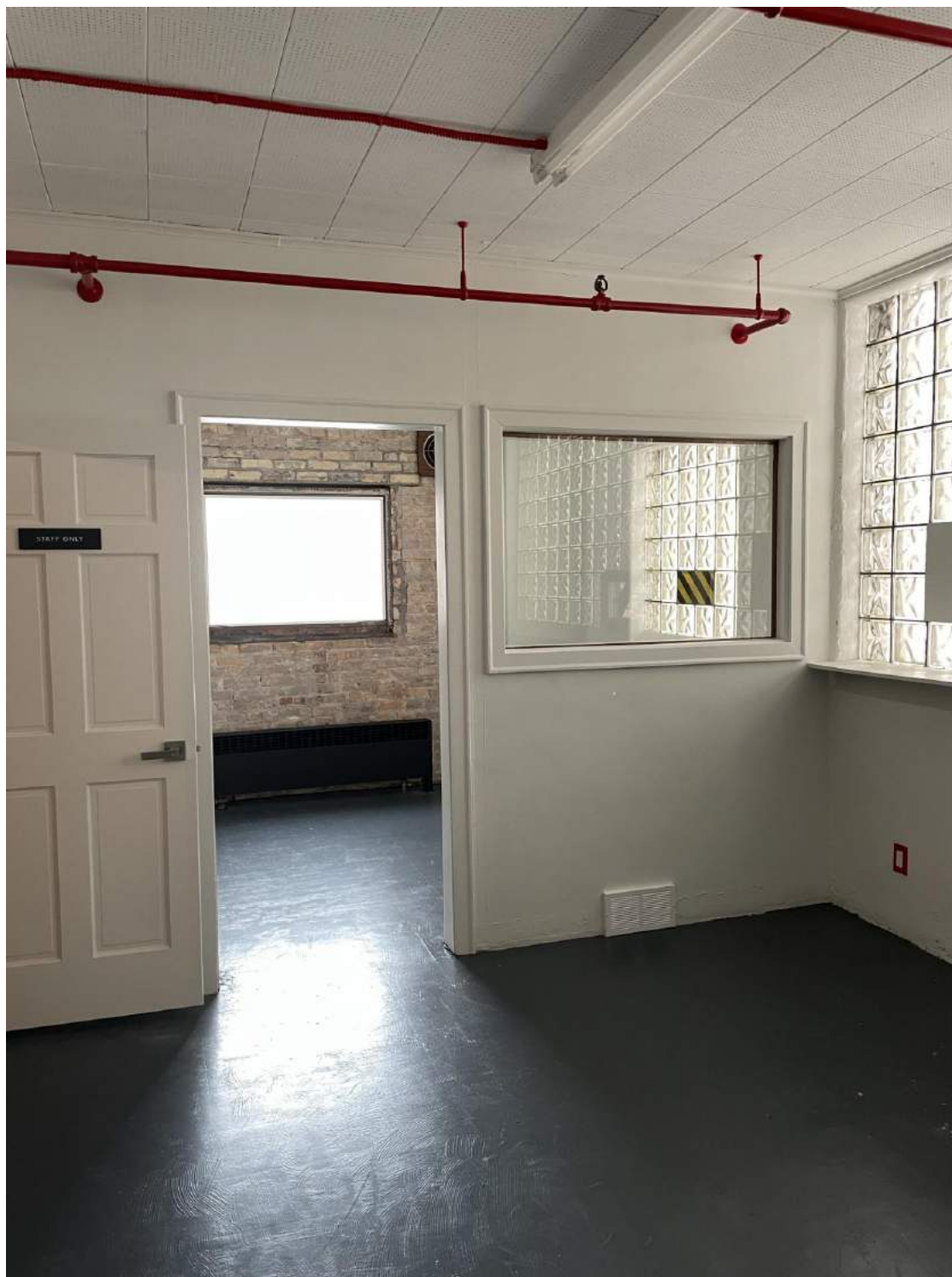
Figure 4.42. Lower Level Office 18W 1 st St, Duluth MN.
