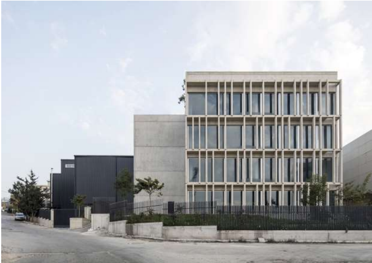
Figure 16 – Yared Warehouse (Khoriaty, 2020)
