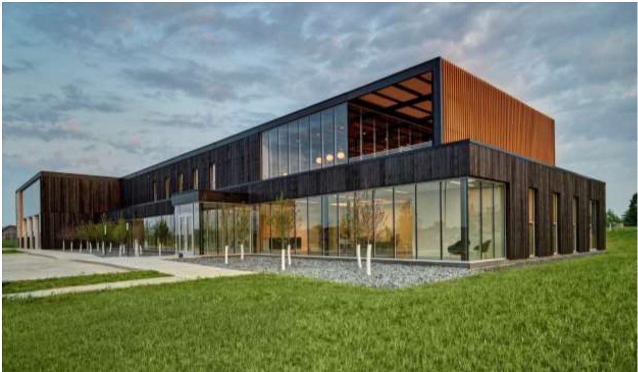
Figure 3 – Marion Fire Station No. 1 (Pintos, 2023)
