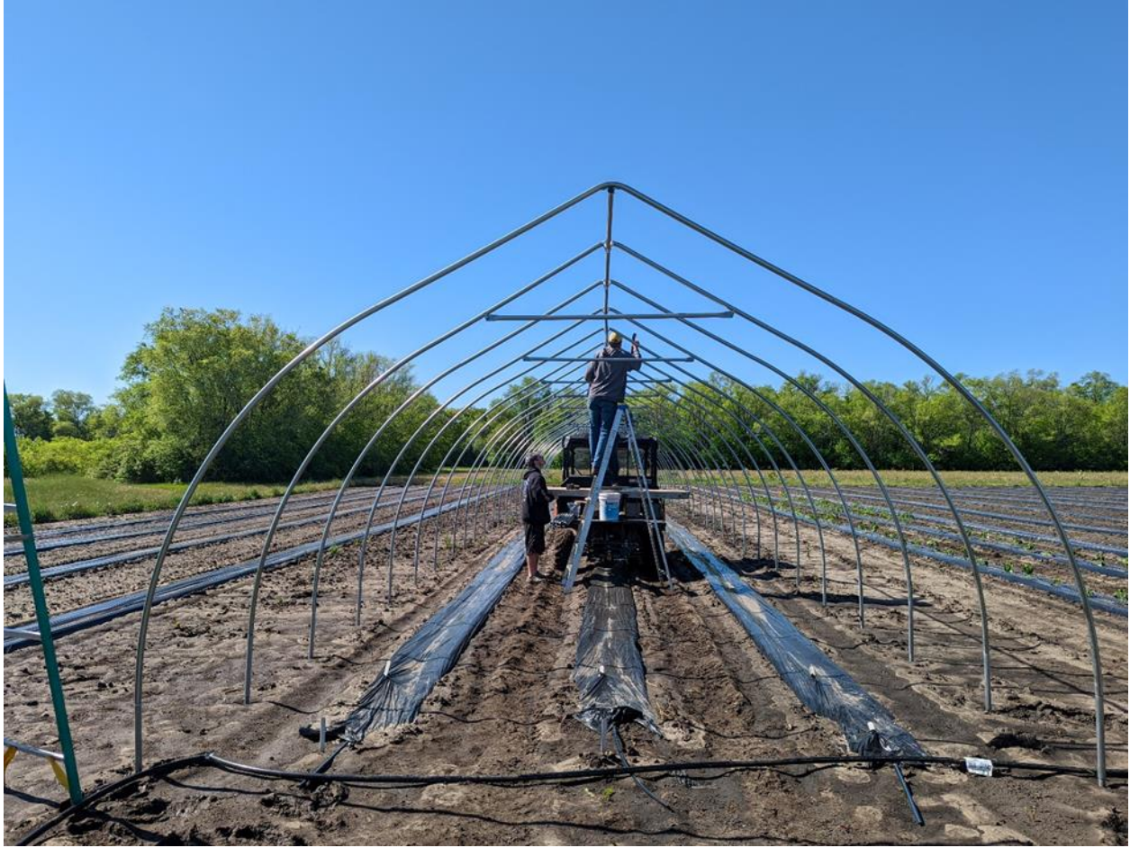
Fig B6. Caterpillar tunnel framing.
