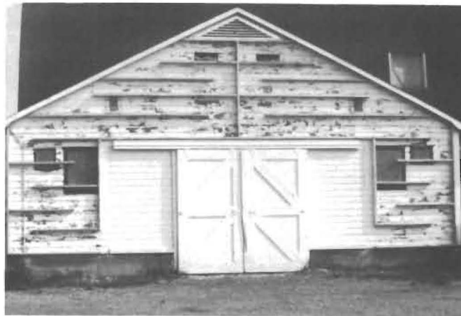
Preparation of the solar collector began with the nailing of 2 x 4's (on edge) to the south wall of the calf housing area of the dairy barn to create air passages.
