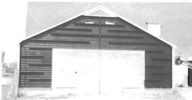
Preparation of the solar collector began with the nailing of 2 x 4's (on edge) to the south wall of the calf housing area of the dairy barn to create air passages.
