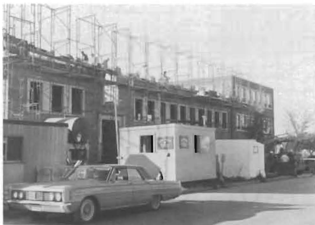
Fig. 2 Addition to Grain Products Laboratory under construction in 1965.
