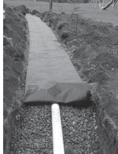
Figure 13. Gravel-filled trench covered with geotextile fabric.
