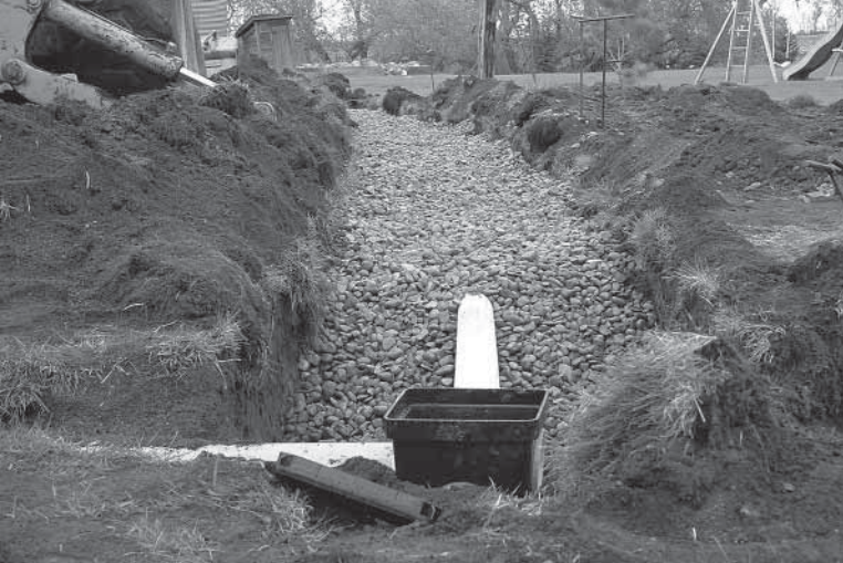
Figure 12. Gravel-filled trench with plastic drop box in the foreground.
