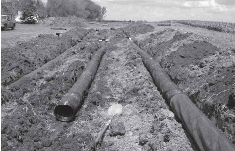
Figure 15. Cylindrical gravelless pipe in shallow trenches. Note the geotextile cover.
