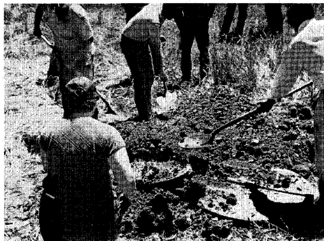
Abandoned wells with diameters of 10 inches or greater are usually plugged with a combination of materials such as sand gravel and native clay. These materials should always be shoveled into the well, as opposed to being dumped rapidly in large quantities.
