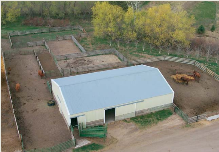
Overhead view of the north barn with outside holding pens, alleys and loading chute on the south side. Barn dimensions are 64 feet by 40 feet.
