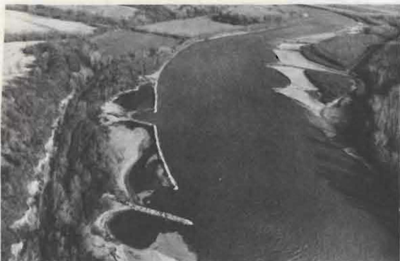
Rulo Bend showing L-head construction above Rulo Bridge.
