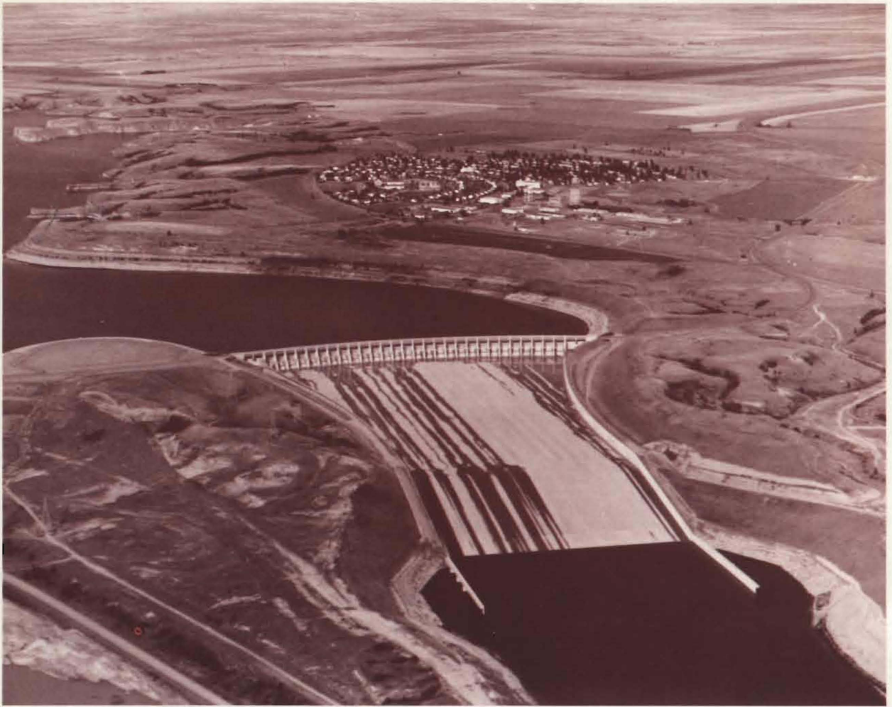
Garrison Dam and Lake Sakakawea provide flood protection not only for North Dakota, but for all of the Missouri River Valley.
