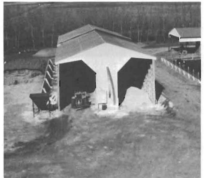
The Solar hay drying shed on the Livestock Unit. Built in 1982, the 42-foot by 100-foot building’s capacity is about 225 tons of hay, and its entire roof is a solar collector. Presently, it’s the site of a series of evaluations of different hay loading systems.
