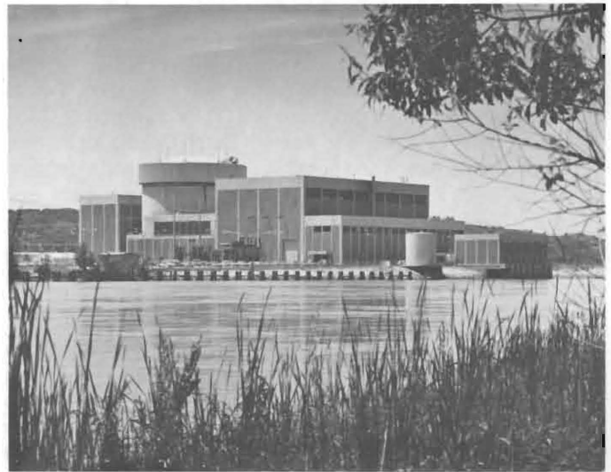
Ft. Calhoun nuclear power plant near Omaha
