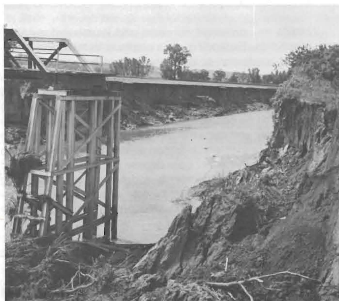
Streambank erosion on Iowa river
