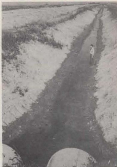
A large drainage ditch in the flat Red River Valley. It carries surplus water to the river.
