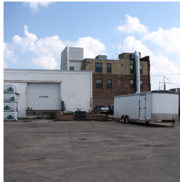
11. Storage west side
