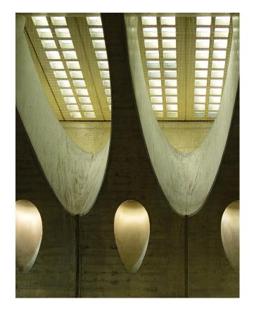
The structure of the railway station is made up of a hallow concrete boxbeam with a covex soffit which replaces the original wall, which is supported by an anchored, piled wall in the rear and by a series of slanted tapering columns in the front. These outstretched arms carry the additional weight of the walkway above, allowing trains to follow the gentle curve of the hillside. (Tzonis, 1999)
