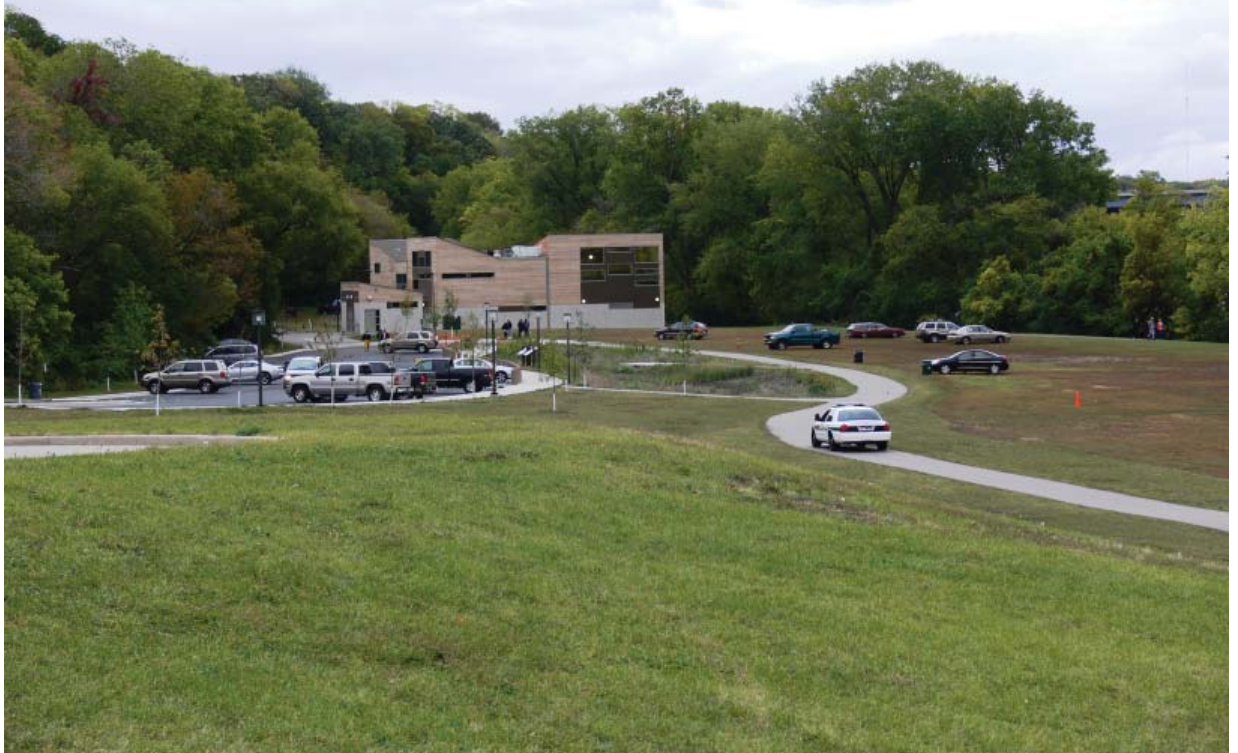
Standing on the west side of the site looking toward the new boathouse
