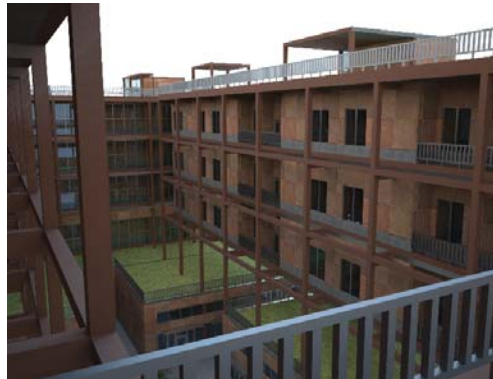
Courtyard View From Bridge
