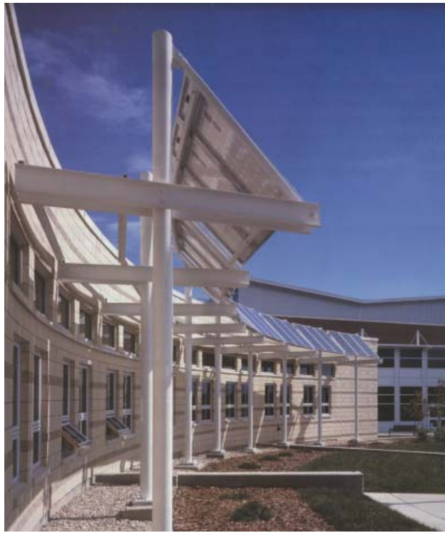
Solar Window Screening Detail
