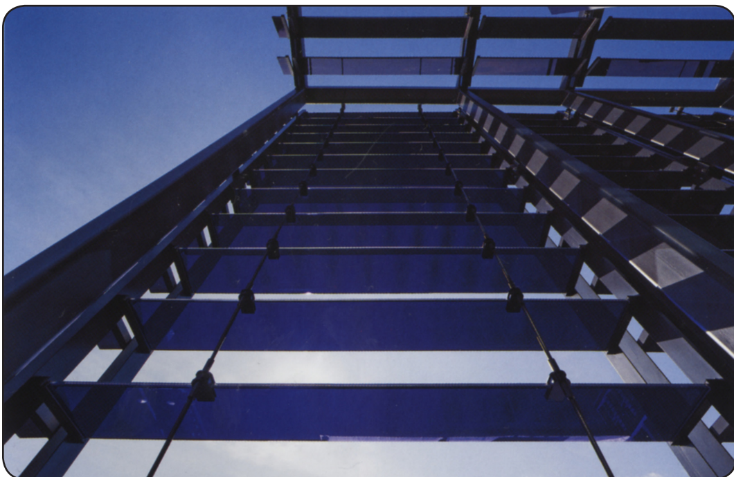
Upward View of Exterior Louvers
