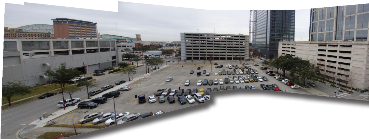
Top of Parking Garage Looking South East |
