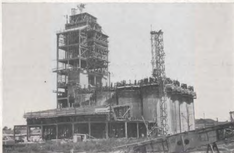
Large cooperative elevator under construction at Rosario.
