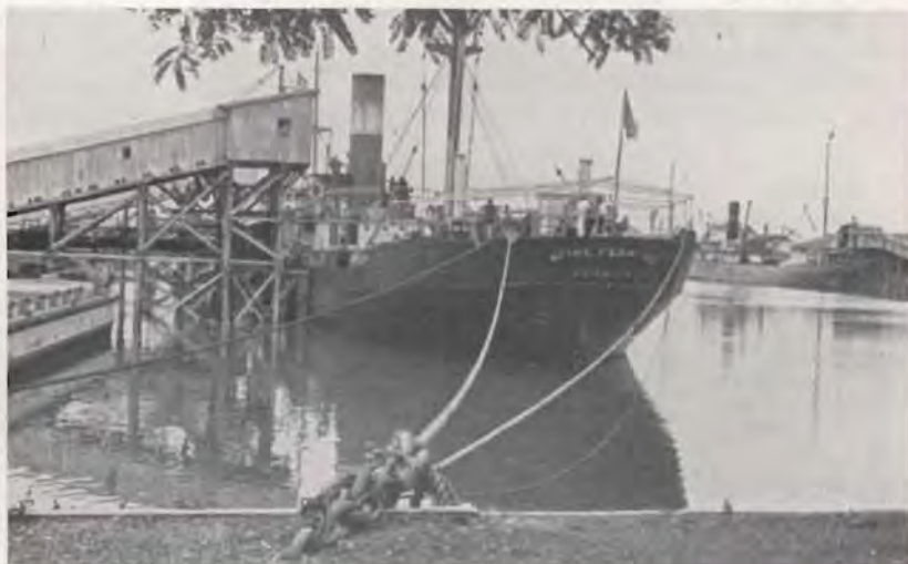
This ocean-going river steamer is being loaded direct from warerooms at Santa Fé. Covered sheds over conveyor belts at this port admit of loading regardless of rain.
