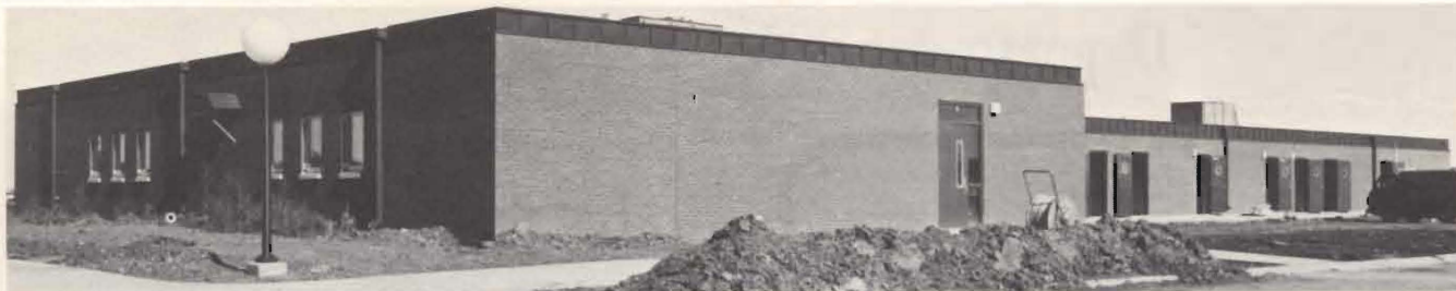
Phase Two of the construction program. This building houses the laboratories and equipment for teaching the new Animal Health Technician curriculum, plus animal isolation units.
