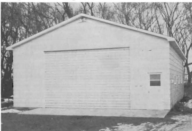
Figure 2. This 32' x 48' farm shop with a wall height of 12'5" and 18' x 12' door opening is considered to be adequate and economical.
