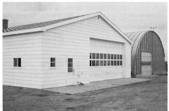
Figure 3. The 36' x 40' x 13.5' size of this farm shop is considered adequate overall, with a 20' x 12' door, but would be hard to heat in winter without good insulation.
