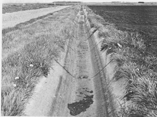
Downslope view to the southeast of the concrete, slip-formed ditch lining.
