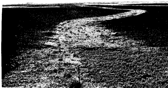
Figure 8 - Small wash-outs should be repaired and reseeded or sodded immediately. Note staggered furrows along waterway edges.
